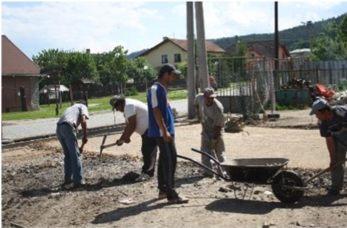
Citizens of Spišský Hrhov during construction works
